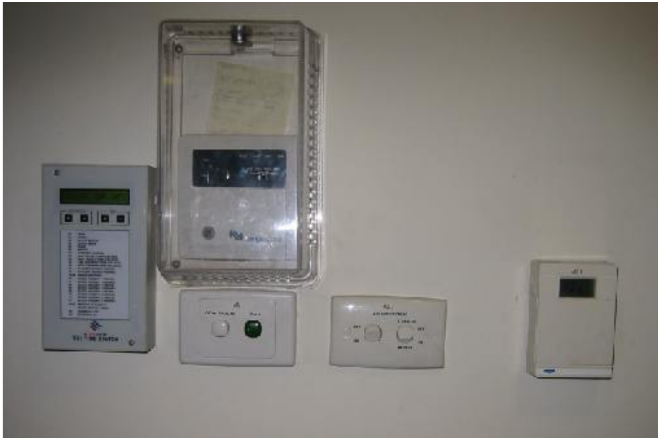
Figure 3 Micro Air TX 1 Time switch, thermostats and after-hours override switches
